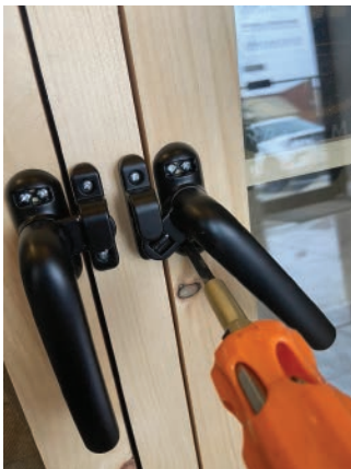
Fasten the right side window handle using 4 screws in the pre drilled locations
