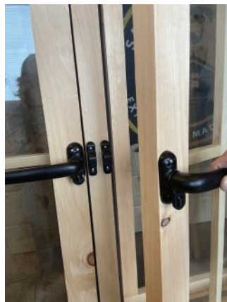
Test window closure and adjust washer height if you need a tighter or looser seal
